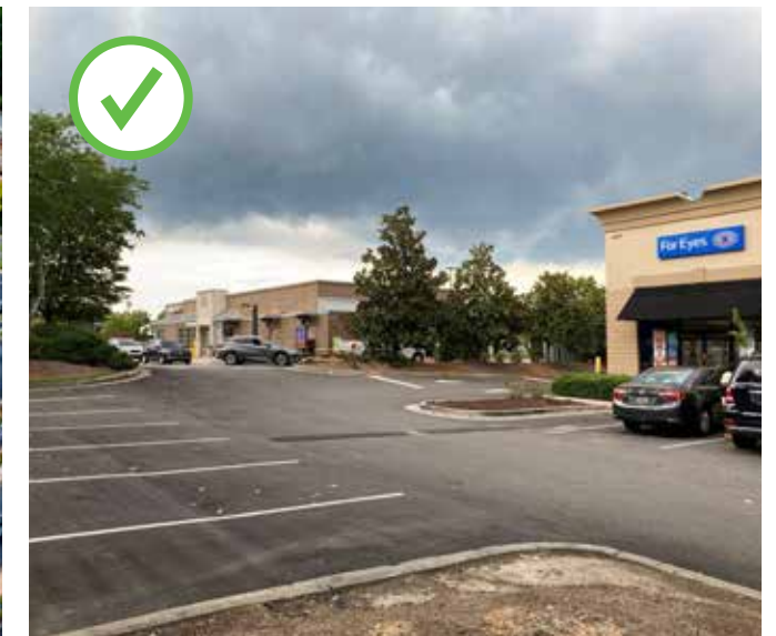
These adjacent commercial developments provide interparcel access to cut down on curb cuts.
