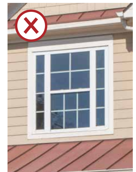
This window is placed flat against the facade, has muntins within the glass, and has poorly designed muntin placement.
