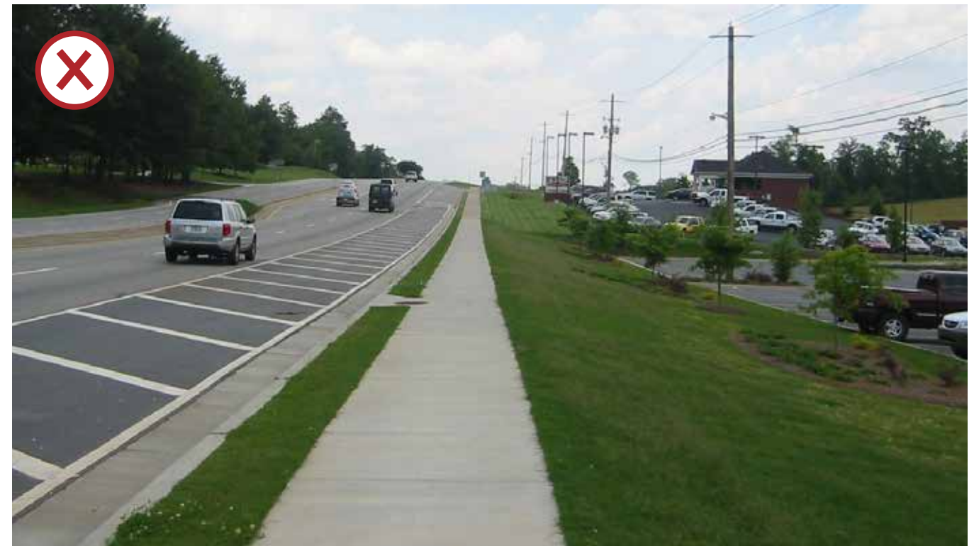
This streetscape has a green strip between and sidewalk and curb, but it isn't sufficiently wide enough to shield pedestrians from traffic.
