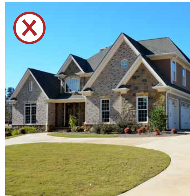
Both types of masonry are combined vertically, with each face having a different material.
