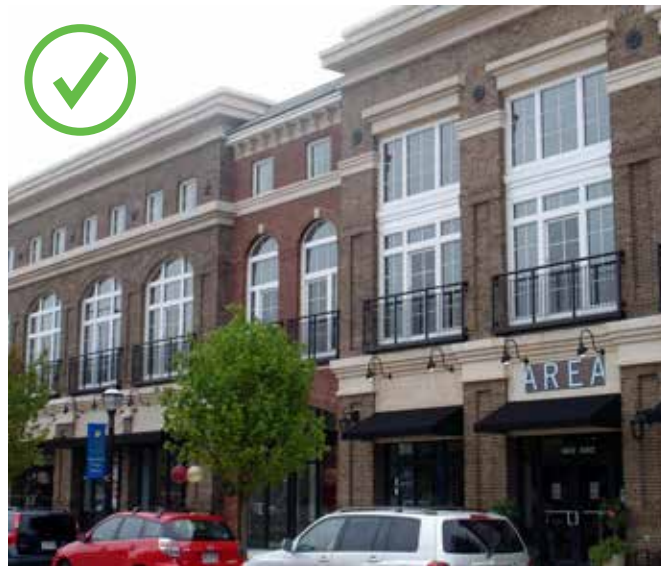
These modules are differentiated through the use of recesses, projections, and articulated bays that create an aesthetically pleasing facade.
