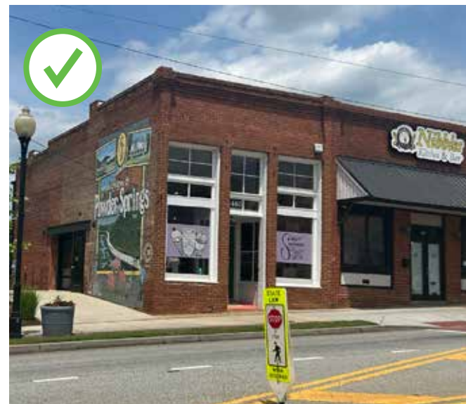
Storefront buildings should feature a lot of glass on their front facades.
