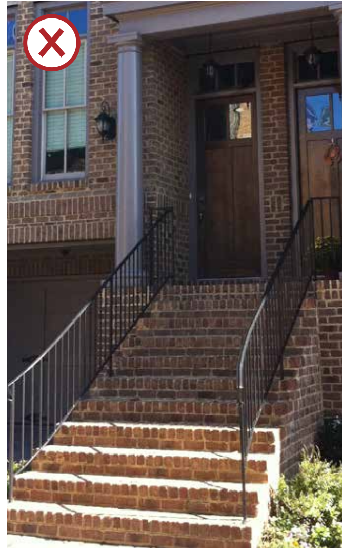
Stoops should not be taller than 6 feet above grade.
