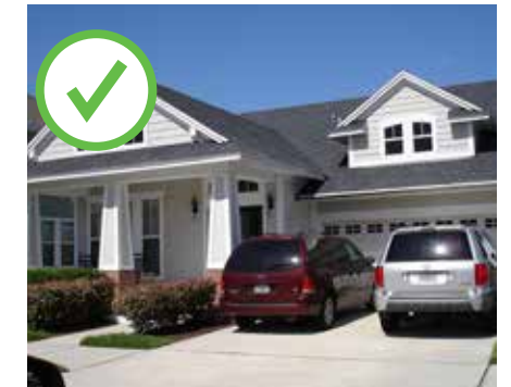
Garages must be recessed at least 10 feet from the main body of the house.
