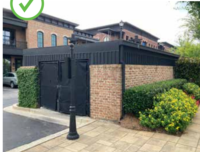
This dumpster screening is compatible with the design of the principal building.
