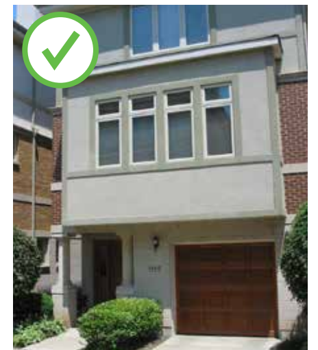
Minimizing the width of garage doors helps to reduce their visual impact.
