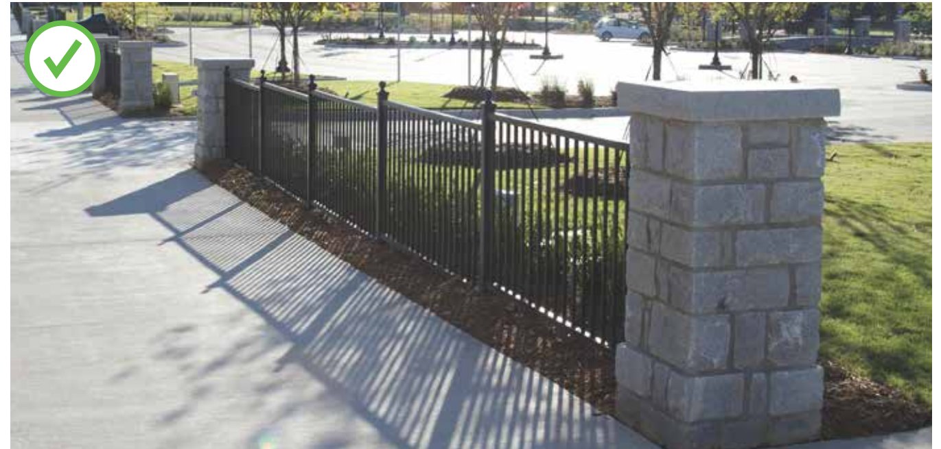
The stone columns on this fence are spaced appropriately.
