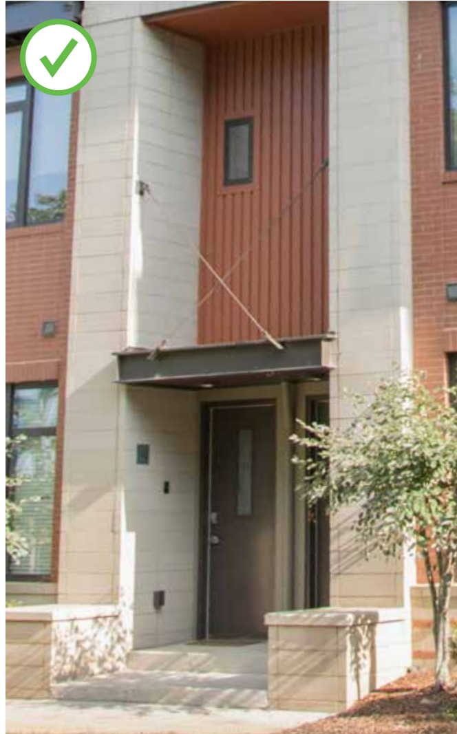
Enclosed stoops are appropriate if they are recessed in the main building.
