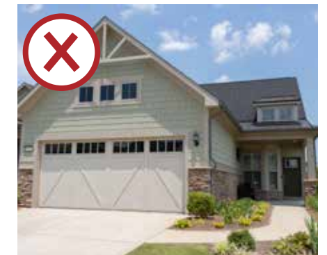
Garages projected beyond the main body of the house should not have the entrance facing the street
