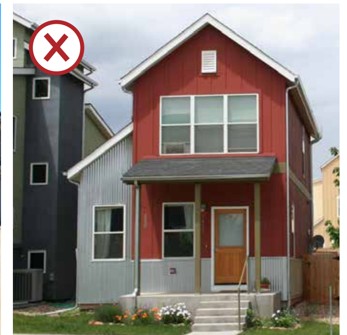
Corrugated metal facades are not allowed.
