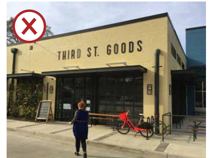
Painted brick is not permitted unless the original brick of the building is damaged and beyond repair.
