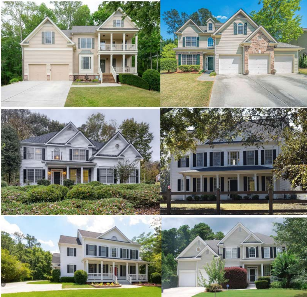
Figure 3. Existing variation from 100% brick elevations.
