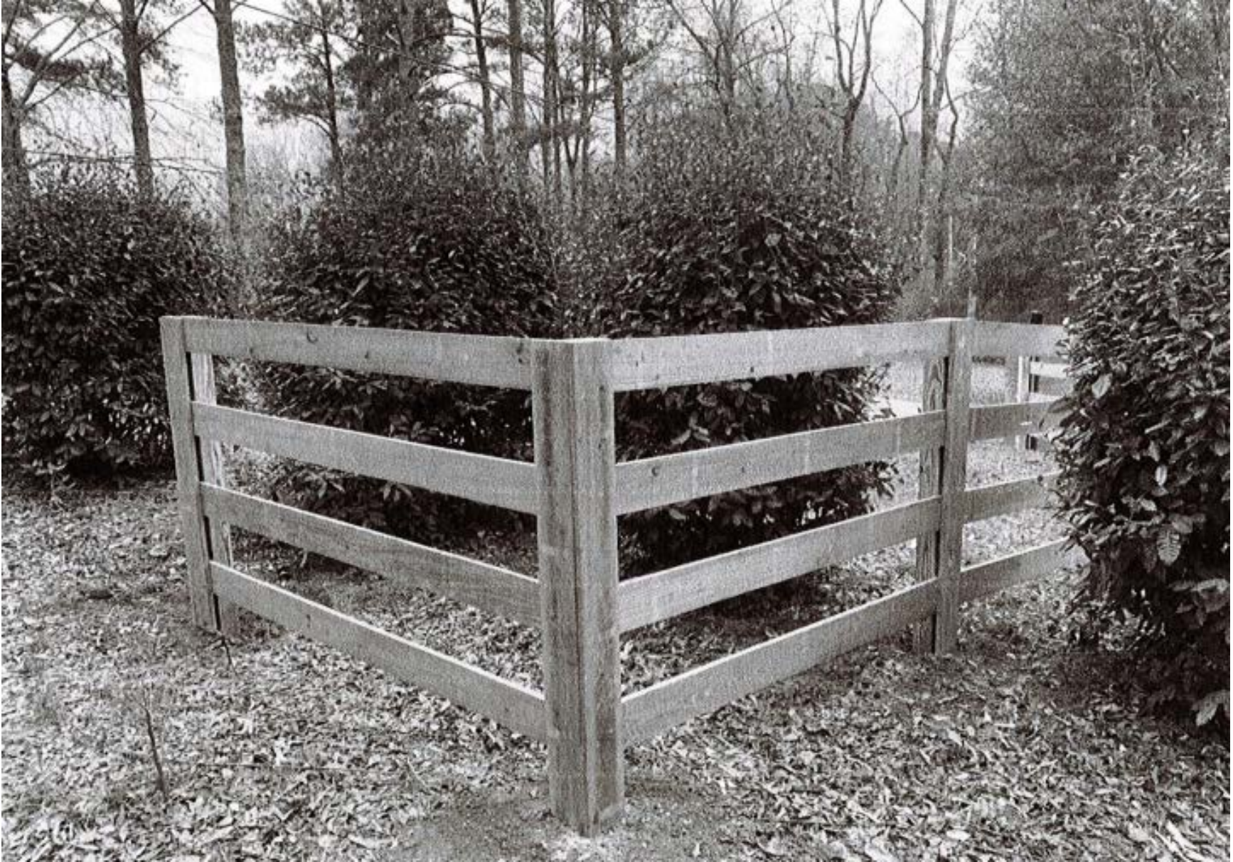
Figure 3. Split rail fence type that the applicant wishes to complete installation with.
