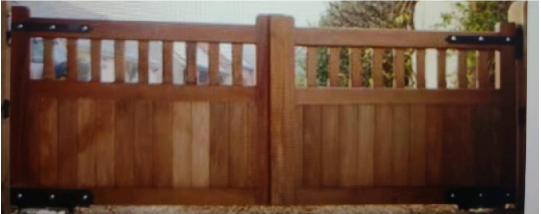
Proposed Gate. The gate is a total of 12' Foot wide with each panel being 59" inches High and 72" inches Wide.
